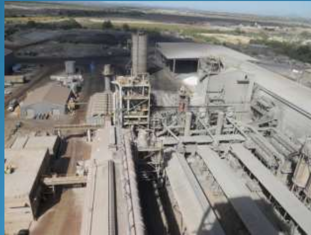
Rillito Cement plant
